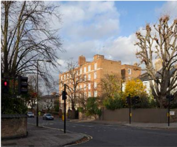
Existing View, looking east from Abbey Road
